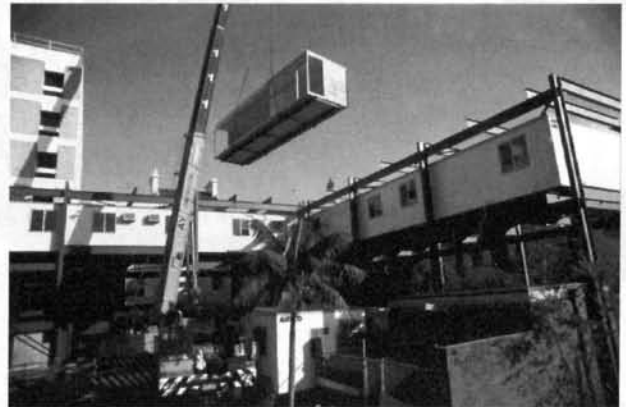
James Hardie Building Systems Ausco office modules are craned into place at the Garvan Institute of Medical Research at St Vincent's Hospital in central Sydney.
